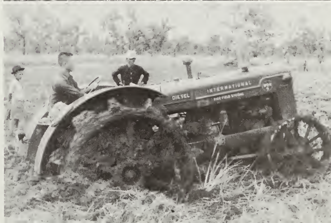
To build a road, they first clear the forest.
